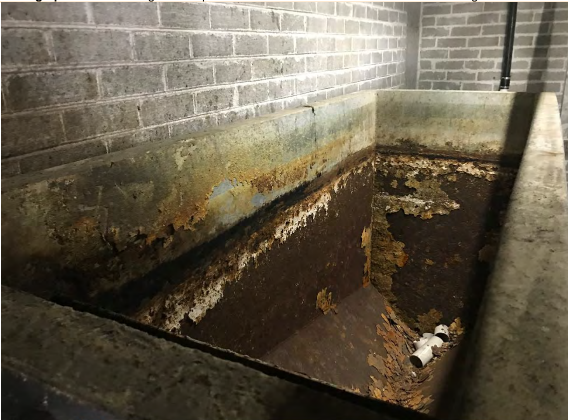
Photograph 14. A disused grease trap observed within the basement level of the building
